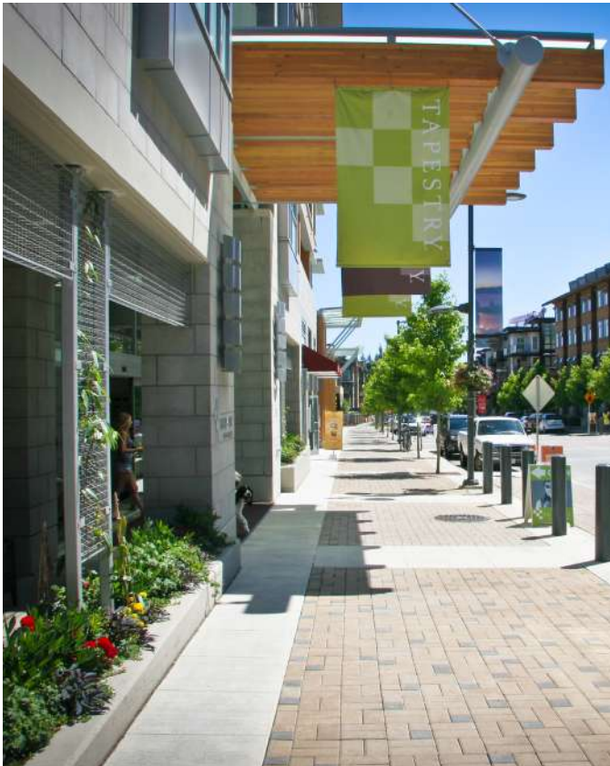
Weather protection at pedestrian entrance to building
