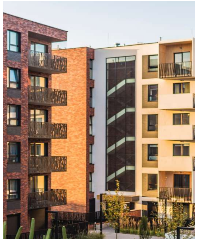
Contrasting approach to materiality
