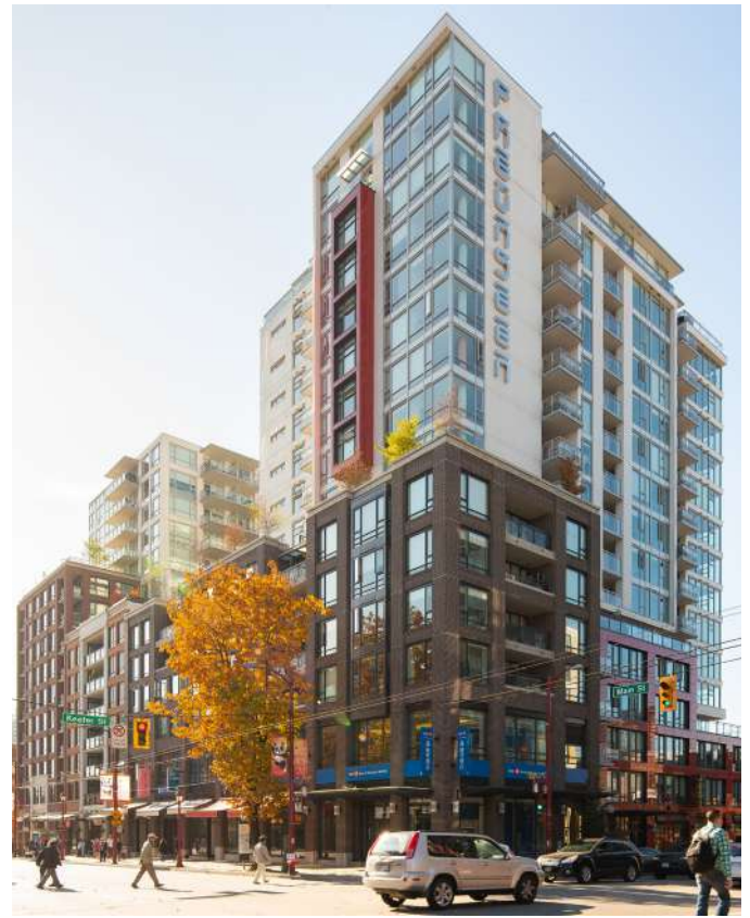
Mixed approach to building articulation and materiality
